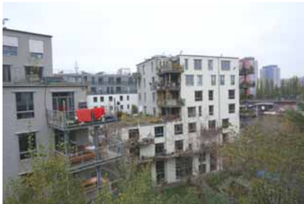
Fig. 08 - Residential buildings (Salma Khamis, 2016)
